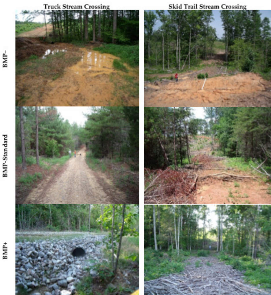
Figure 1. This image from Nolan et al. 2015 shows the real impacts that BMPs can have on stream crossings. BMP- (top photos) delineates crossings that are not meeting BMPs, and the accompanying images show an extremely degraded crossing that will contribute significant sediment to the stream. BMP-Standard (middle photos) indicates that BMPs are met and BMP+ (bottom photos) indicates that those BMPs are exceeded. The likely decrease in sedimentation from these latter two categories is clear in the accompanying images.
